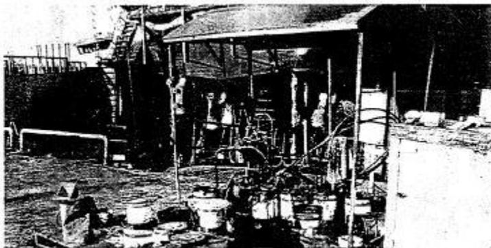
**Portable shelter for paint mixing with rain cover and recessed metal floor for containment.**
